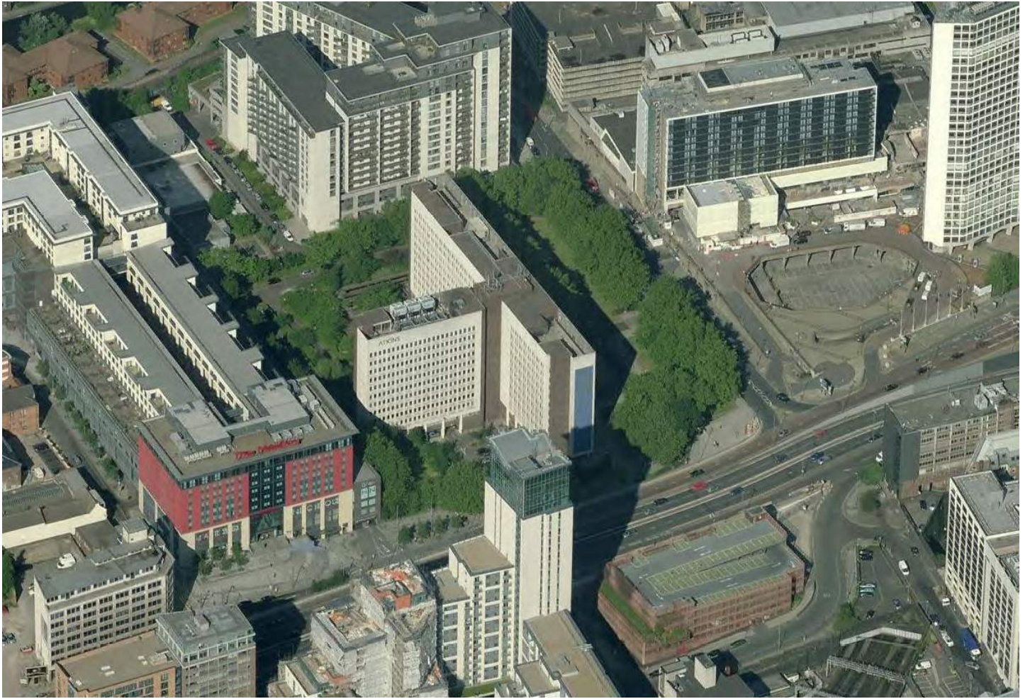
Photo 2 – Wider ariel view of the existing building and its context
